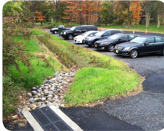
In developed landscapes, stormwater runoff from parking lots, driveways, sidewalks, and rooftops flows to drainage pipes that feed the sewer system. The cumulative effect of these impervious surfaces and thousands of connected downspouts reduces the amount of water that can infiltrate into soils and greatly increases the volume and rate of runoff that flows to waterways.
